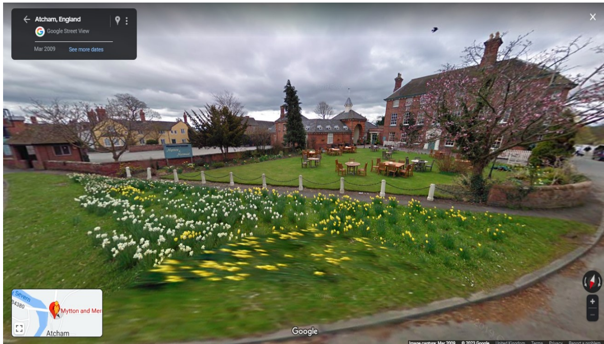
- Front view of the premises from B4380 -
